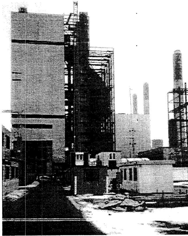
Nordjyllandsvaerket Project with completed SCR
